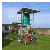
Drinking Water Supply
